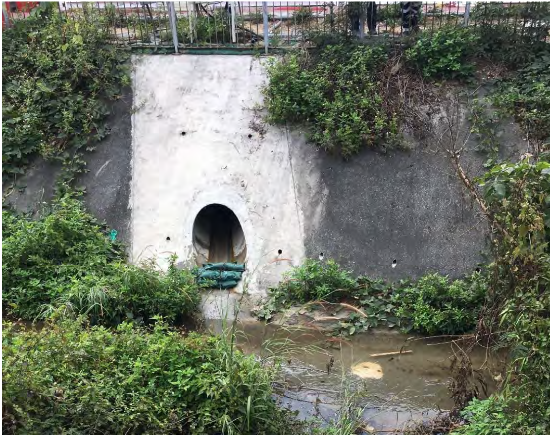
Sand bags were provided at the stormwater terminal discharge point.
