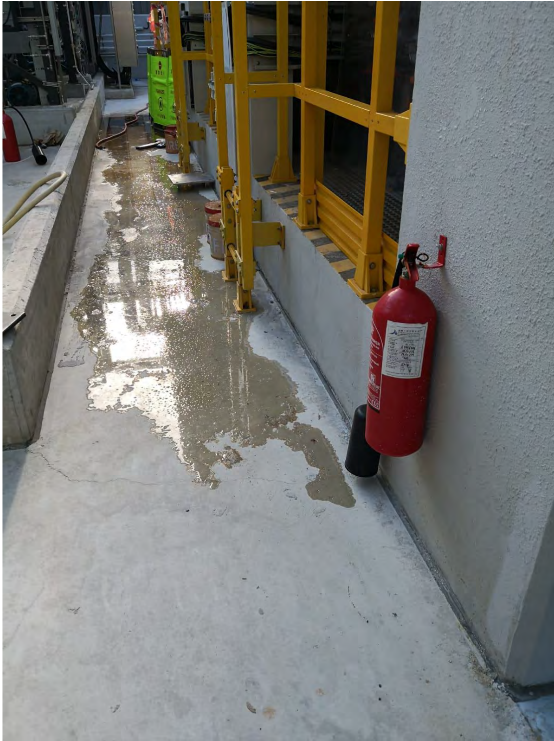
Chemical leakage observed on Building 1 roof.
